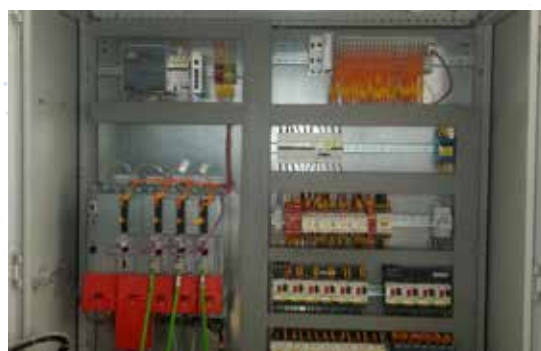
Control cabinet with a PLC controller and SERVO inverter
